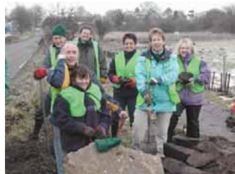
PKF spend a day rebuilding drystone walls at Markfield
